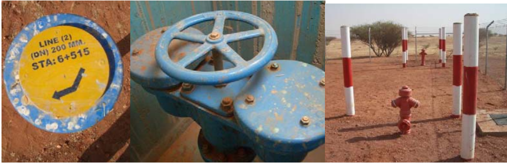
pipeline marker post (c r), line vent (d l), fire hydrants (d r)
