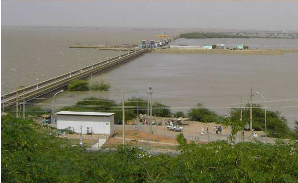
White Nile at potable water transmission line White Nile crossing(d), ground water line PVC DN200 (8") (t)
